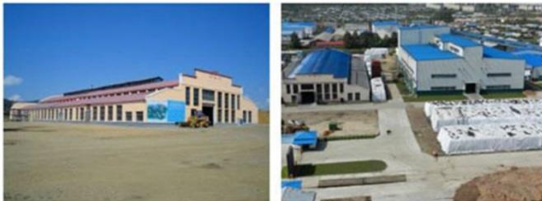
Facilities of Tahe Biopower Plant
